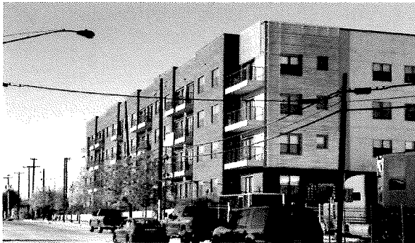
Maple Station – 5522 and 5602 Maple Avenue
