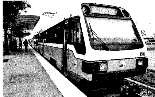
Deep Ellum Light Rail Station
