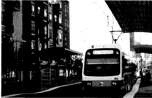
Baylor Light Rail Station
