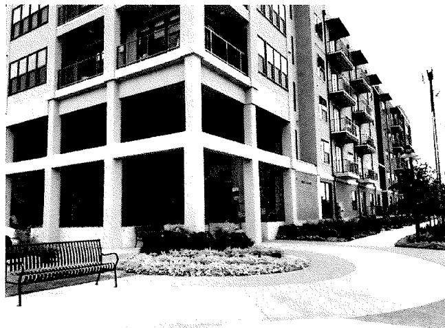
Alexan Riveredge, completed 2017
