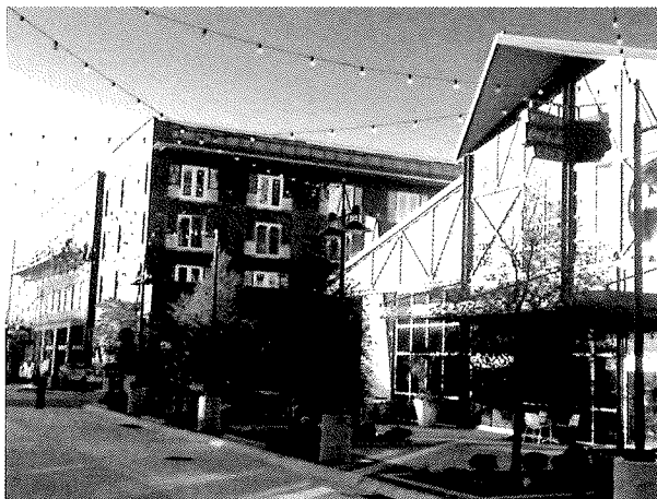
Street view between Taylor Building and Farmers Market Shed 2 Harvest Lofts (Shed 3 and 4) in distance
