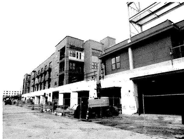
Taylor Street construction
