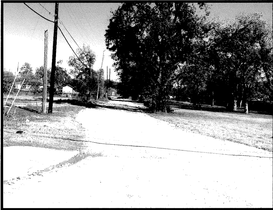
Looking north along Meek Street from Carbondale Street
